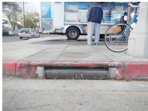
Current drainage catch
