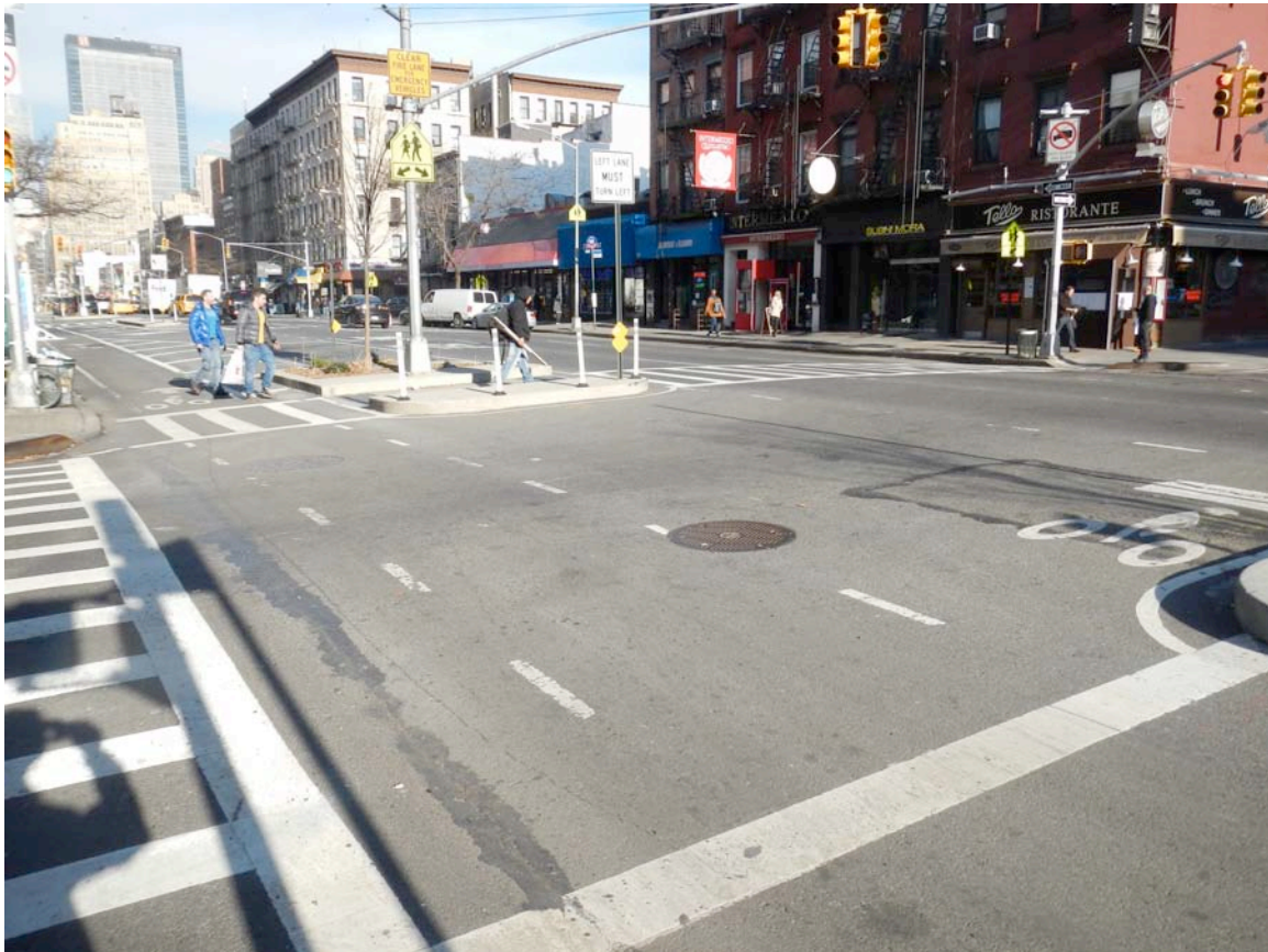
Example of Street with Protected Bike Lanes. Notice Pedestrians using the oasis.
